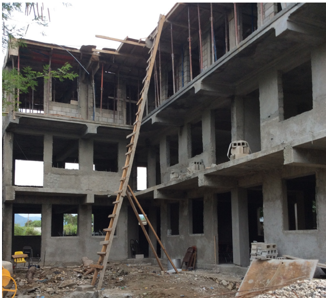
Secondary building nears completion at HAC.
